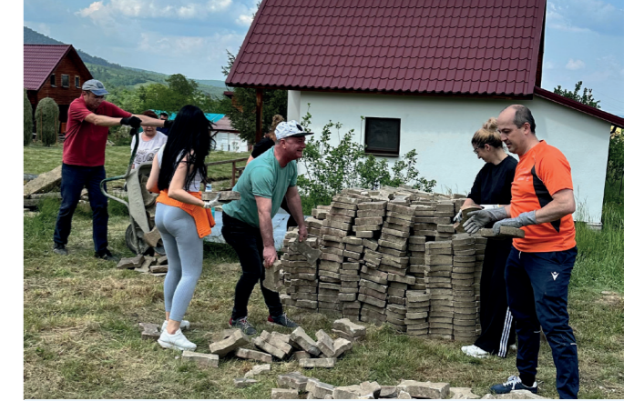
Our team in Romania dedicated time to help renovate properties at Motivation Camp, an initiative supporting people with disabilities in learning how to adapt to using their motorised wheelchair.
